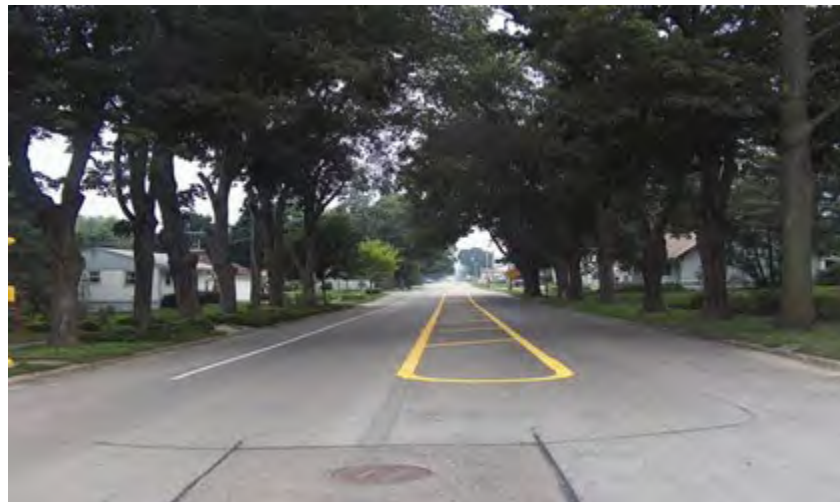
Figure 6.9 Wide centerline median striping.
