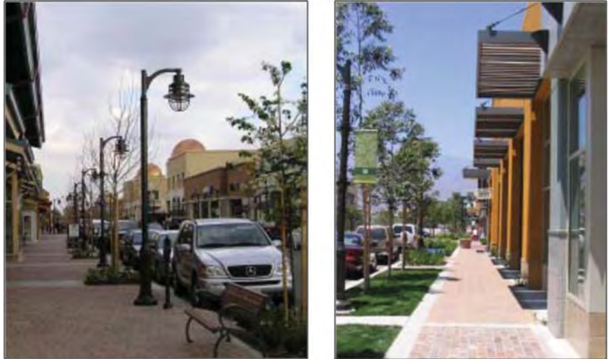
Figure 5.45 Street trees centered in extended paved surface and in a tree lawn.
