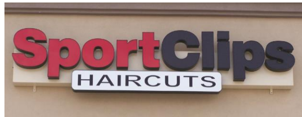
Discouraged – Exposed Raceway
