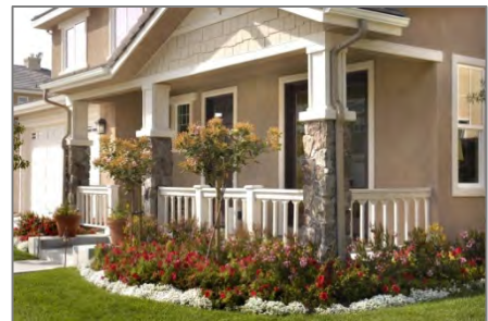
Figure 5.14 Front porch scaled appropriately.
