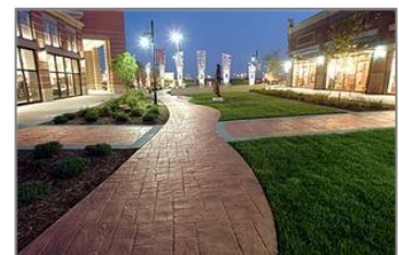
Figure 5.54 Stamped and stained concrete.
