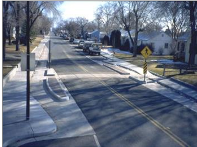
Figure 6.7 Chokers on a residential street.
