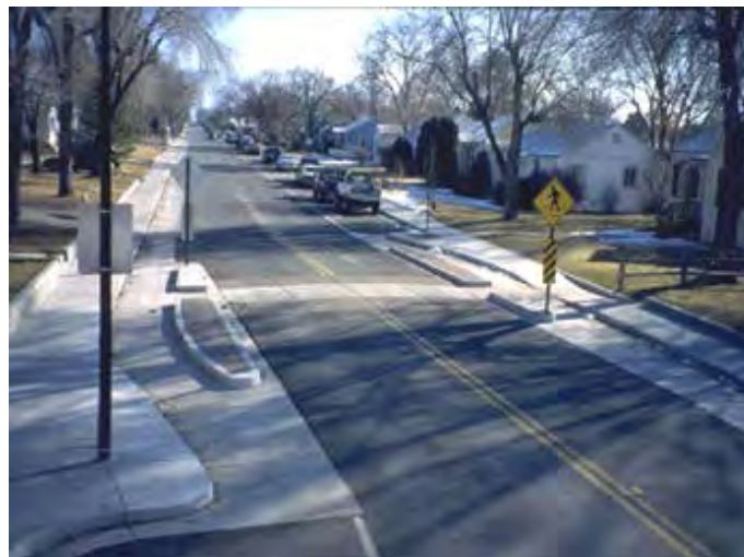
Figure 6.7 Chokers on a residential street.
