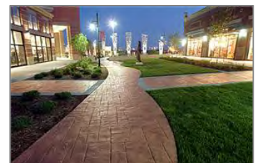
Figure 5.54 Stamped and stained concrete.
